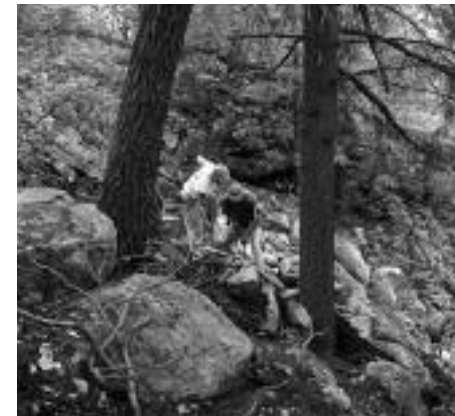
Completing rock work on the Gertrude's Nose Trail in Minnewaska S.P.
