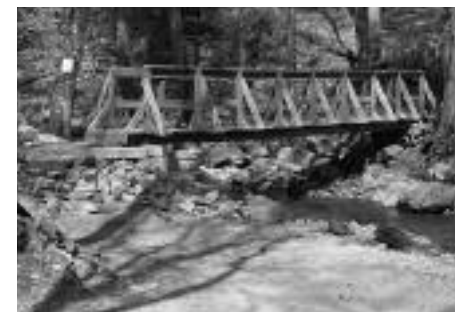
The new bridge over Dunnfield Creek. See an illustrated chronology of the project at http://www.trailstobuild.com/gallerys/dunnfield_creek.htm
