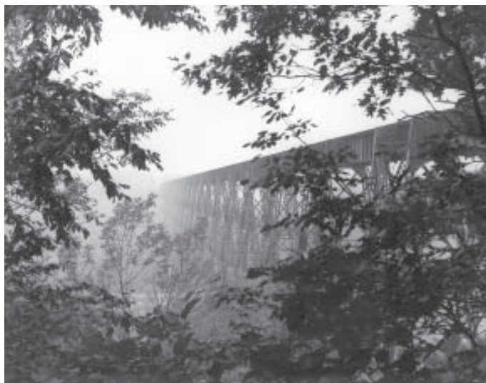
The Moodna trestle, as seen from the Trestle Trail
